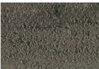
DRIVEWAY (NSW): COLOURED CONCRETE
