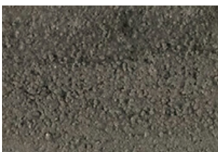
DRIVEWAY (NSW): COLOURED CONCRETE
