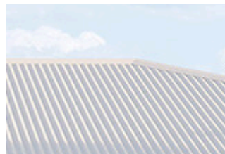
COLOURBOND ROOF: DOVER WHITE
